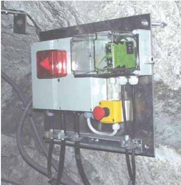
Figure: Compact flashing light used for a safety application in a tunnel. The input voltage range of 70–264 V AC and 73–140 V DC supports both line (mains) and backup battery power
