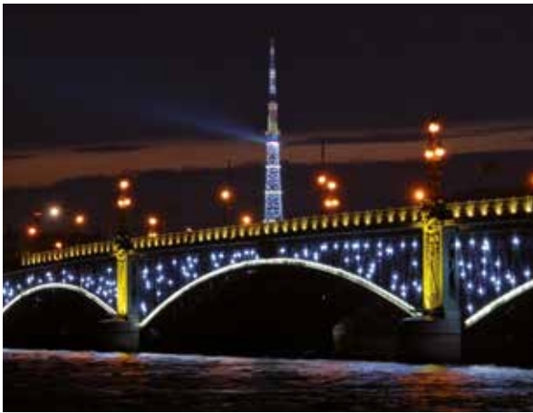
St. Petersburg, Russia TV Tower and Trinity Bridge 9,500 Pfannenberg flashing lights
