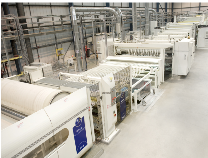
BHS Corrugated Dry End
