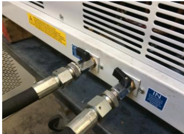
Picture 11 – Pipe connection
