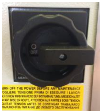
Picture 8 – Main switch
