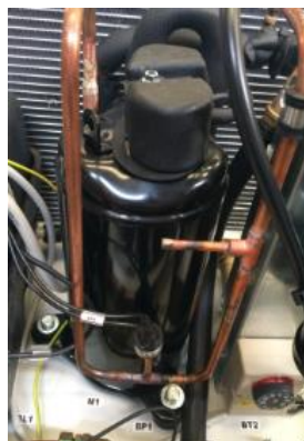
Picture 16 – Compressor placement
