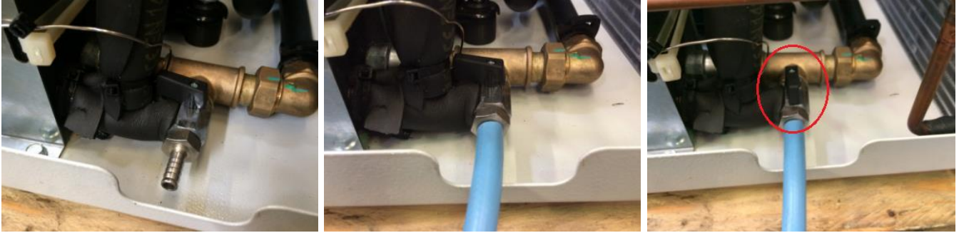
Picture 22/23/24 – Chiller draining
