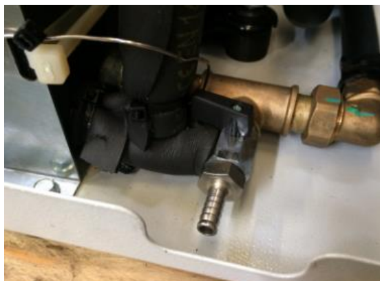
Picture 5 – Hydraulic draining connection
