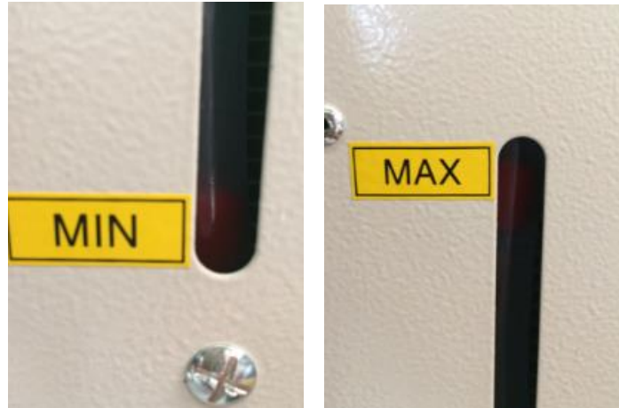
Picture 13/14 – tank top up
