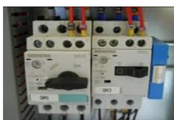
Picture 8 – Circuit breakers
