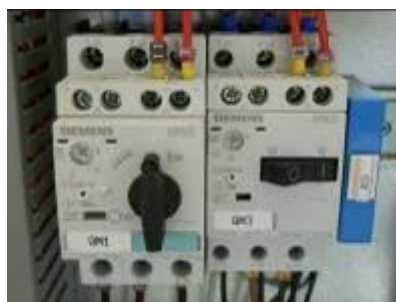
Picture 20 – All circuit breakers ON
