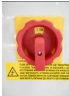
Picture 17 – Main switch ON
