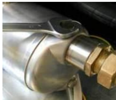
Figure 15 – Purge de la pompe
