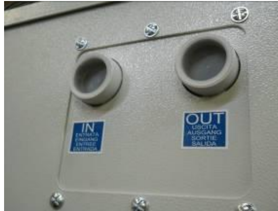
Picture 3 – Hydraulic connection plate
