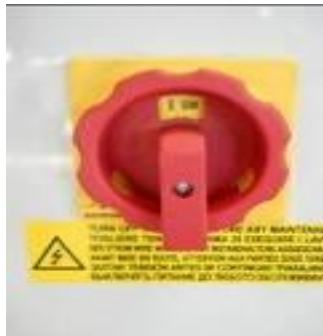
Figura 17 – Interruptor general en ON
