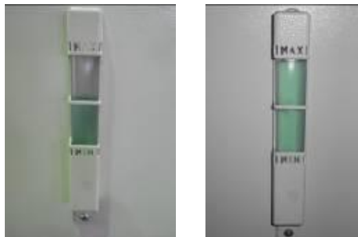
Picture 18 / 19 – Tank top up
