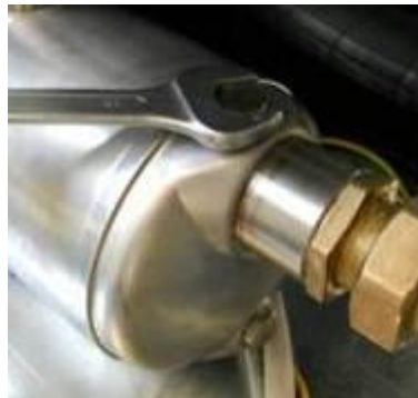
Picture 15 – Pump purging
