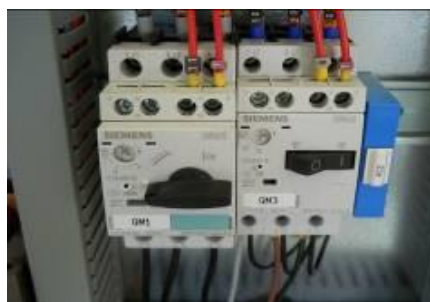
Picture 16 – Pump breaker ON
