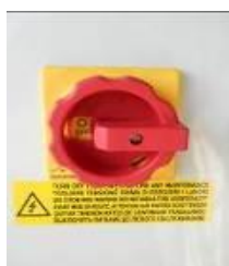
Picture 7 – Main switch
