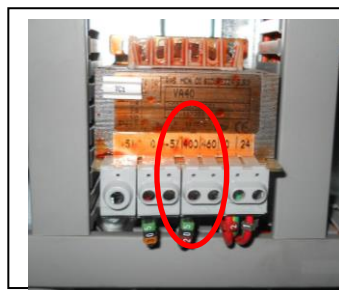
Picture 5 Transformer set at 400V
