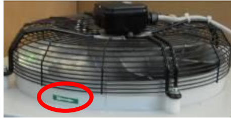
Picture 21 – Fan rotating direction
