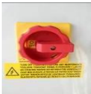
Figura 7 – Interruptor general OFF
