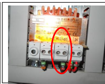
Picture 6 Transformer set at 460V
