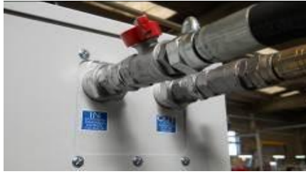
Picture 13 – Pipe connection
