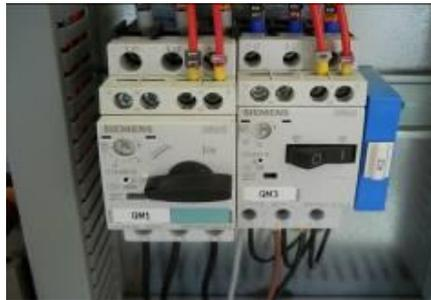
Picture 16 – Pump breaker ON
