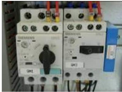
Picture 20 – All circuit breakers ON
