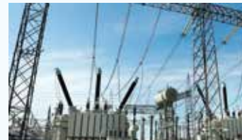
Energy generation and supply
